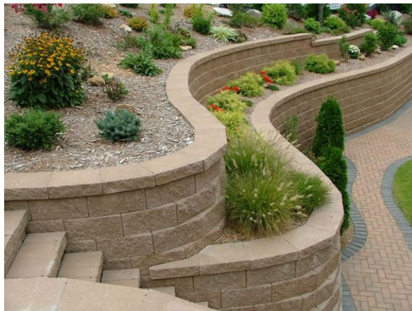
Figure 19: Retaining walls shall be benched, or terraced, so that no individual wall exceeds a height of six feet.
