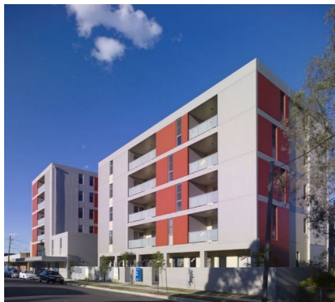
Figure 13: Illustration showing recessed or flush balconies
